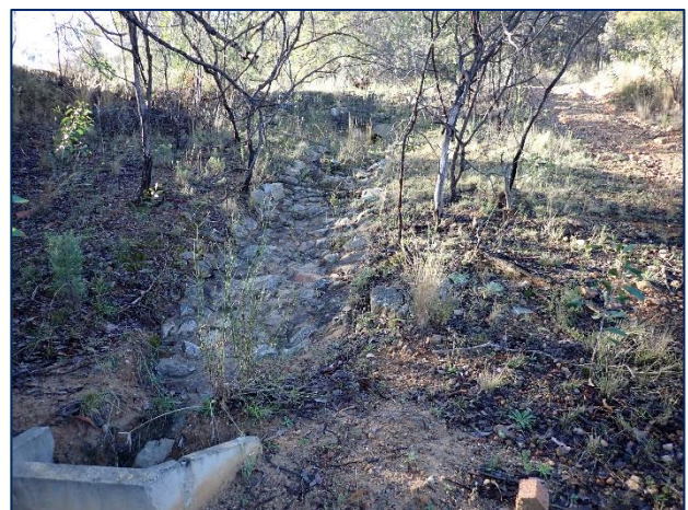
Photo 4-6: View east of concrete-and-rock drain adjacent to water reservoir fence.
